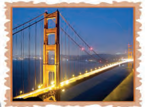
Golden Gate Bridge, San Francisco
