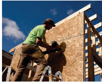
Mason builds our house
