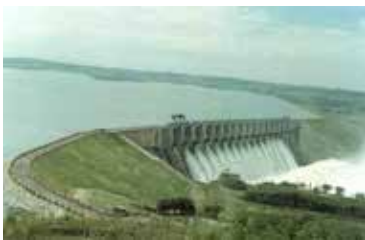
Work going on at the Gandhi Sagar bandh (completed in 1960)
