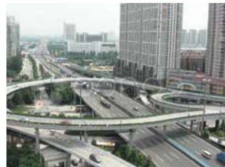
Road Network with flyovers
