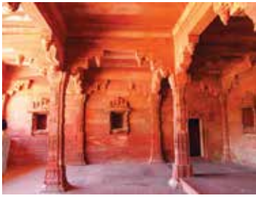
Pillars and struts holding the extension of the roof in Jodha Bai Palace in Fateh Pur Sikri.
