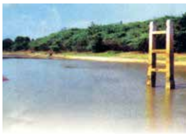
A ninth-century sluice gate in Tamil Nadu
