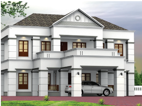
House with sloping roof
