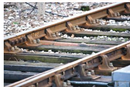
Gaps for expansion between two sections of rail tracks
