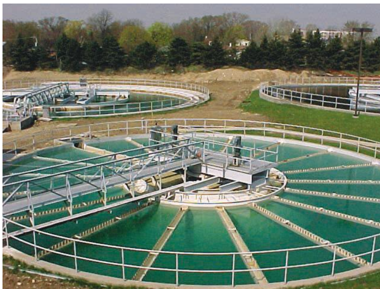
Water treatment project
