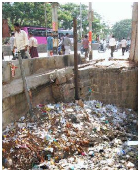
Open drainages, a serious health hazard
