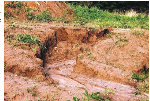
Soil erosion by rain
